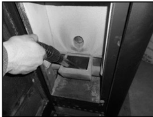
Figure 17 - Interior cleaning
